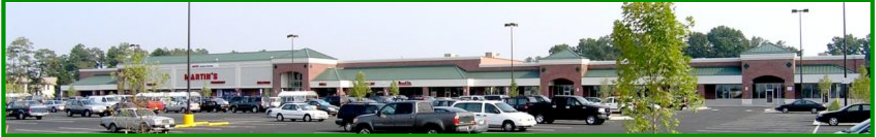
Fredericktowne Crossing: Martin's Grocery Store and Other In-Line Retails
